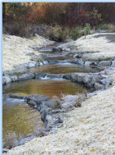
Figure 7: Step Pools at the Chumstick Creek 2010 Restoration Project
