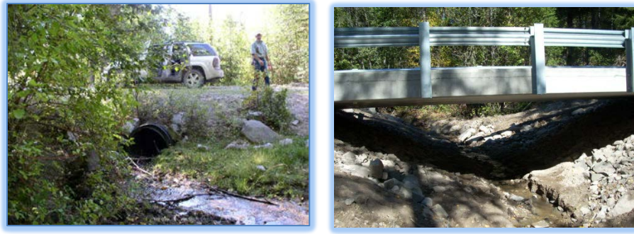
Figure 4: Before and After at an Upper Omak Creek Culvert Replacement
